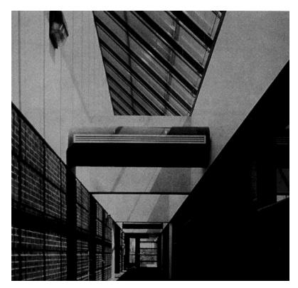
Figure 1-7: Direct Gain plus Storage. Air National Guard Composite Operations and Training Facility, Bangor, Maine
