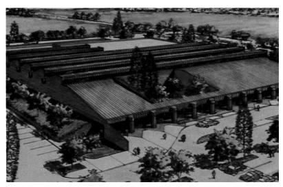
Figure 1-24: Monitor Apertures. Commissary, Vandenberg AFB, California
